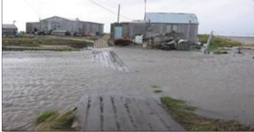
Figure 14 Flood in Alaska Native village of Newtok. Image sourced from Alaska Department of Environmental Conservation.
